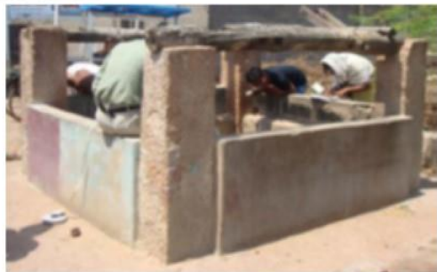
Revival of old unused well for decentralized piped supply for a slum
